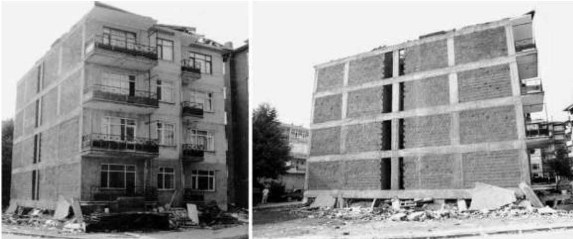
Figure 7. First two stories collapsed building – Kocaeli earthquake (photos by K. Mosalam)
